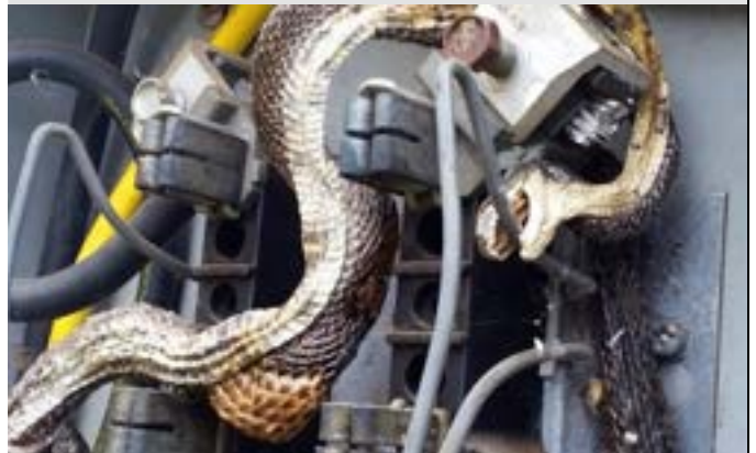
Pests and their predators can be attracted to warm, dry spaces inside transformers
