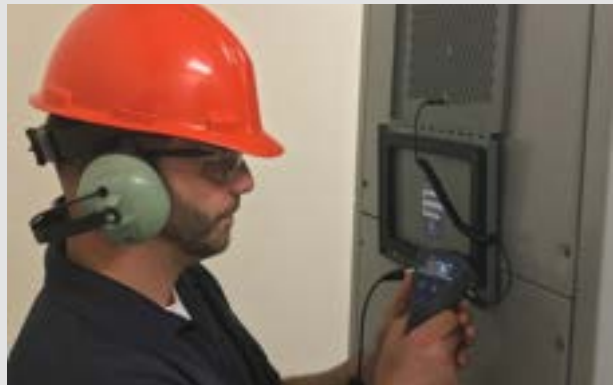
With a maintenance inspection window for visual, infrared, ultraviolet, and ultrasound inspections installed on medium voltage switchgear, no special PPE is required to use the EMSD
