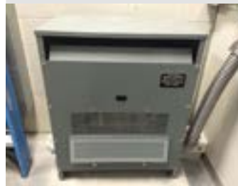
Custom replacement dry transformer panel-front with a built-in maintenance inspection window
