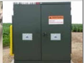
One large format maintenance inspection window is fitted on the LV side and another on the HV side of an oil-filled pad mount transformer allowing for inspection of all the internal connections
