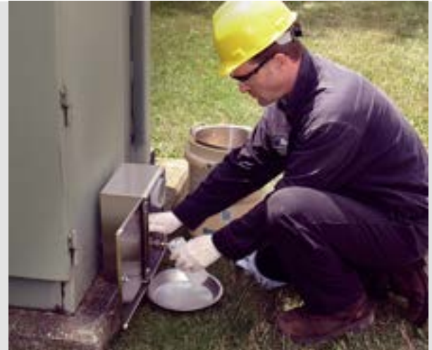
A safer oil sampling method retrofitted to an existing transformer allows energized sample collection; the sampling cabinet is lockable to prevent unauthorized access (Courtesy SDMyers)
