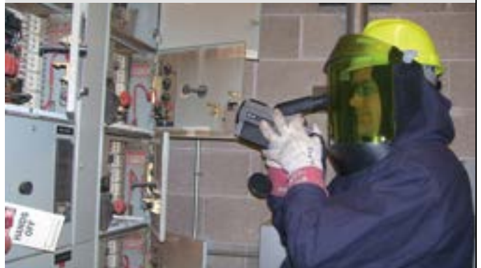
Infrared scanning is applicable on all electrical assets including motor control centers, but typically requires extensive PPE if done “open panel”
